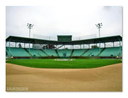
The wooden grandstand was replaced by a steel and concrete structure in 1949/50, increasing seating capacity to over 3,500 spectators.
